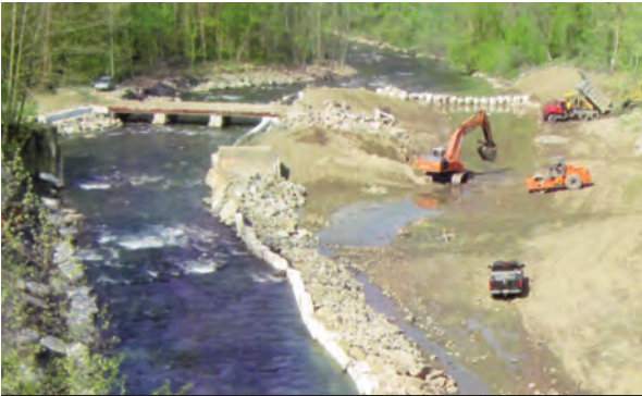
Union Dam Demolition Design and River Channel Restoration Gannett Fleming Inc.
