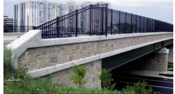
MD 355 Interchange Design Build KCI Technologies Inc.
