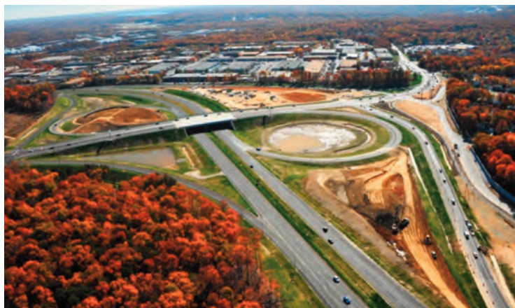
Johnson, Mirmiran & Thompson Fairfax County Parkway Design-Build (Fort Belvoir, VA)
