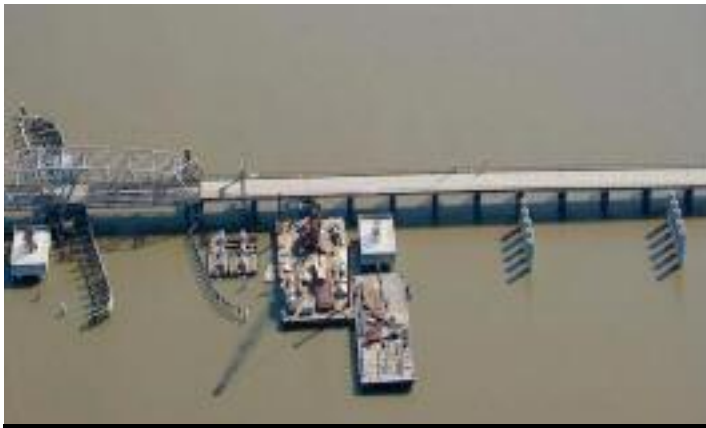
Honor Award - Alvi Associates Fender / Dolphin Systems for Route 5 Bridge over Chickahominy River
