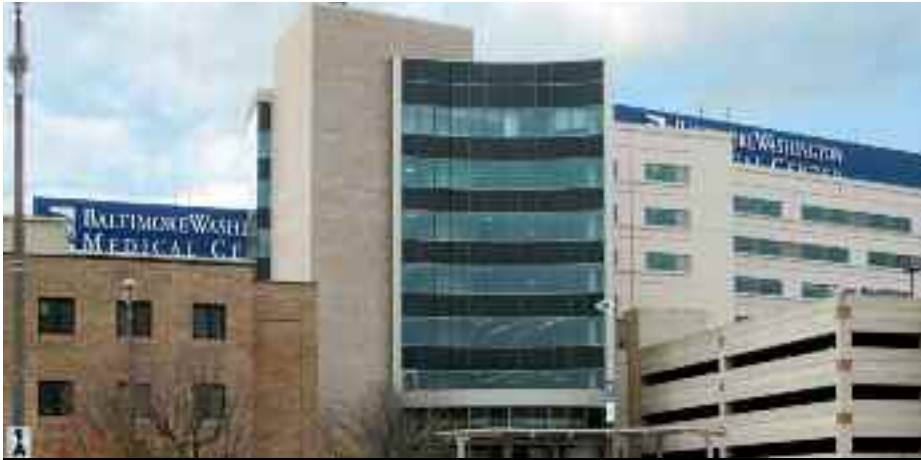
OUTSTANDING PROJECT AWARD IN STRUCTURAL SYSTEMS - Inpatient Tower & Women's Center at Baltimore-Washington Medical Center (Glen Burnie, MD) - WBCM
