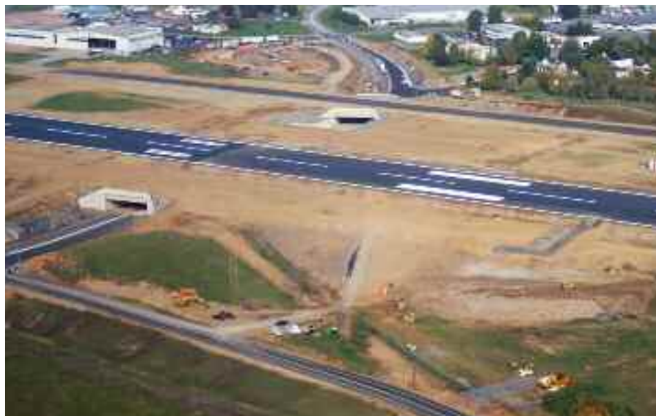
OUTSTANDING PROJECT AWARD IN SPECIAL PROJECTS - Runway 9-27 Extension and Associated Improvement (Hagerstown, MD) - URS Corporation
